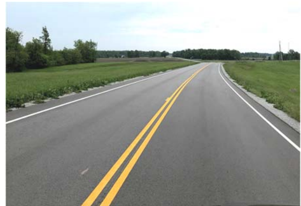
County Road 304 - After Resurfacing
