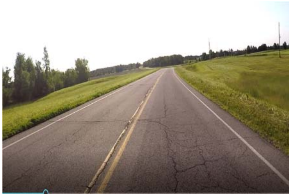
County Road 304 - Prior to Resurfacing
