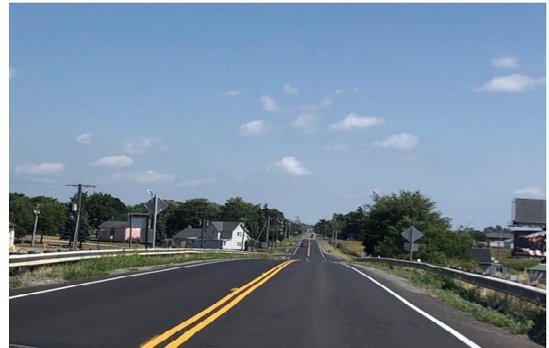
County Road 313 - After Resurfacing
