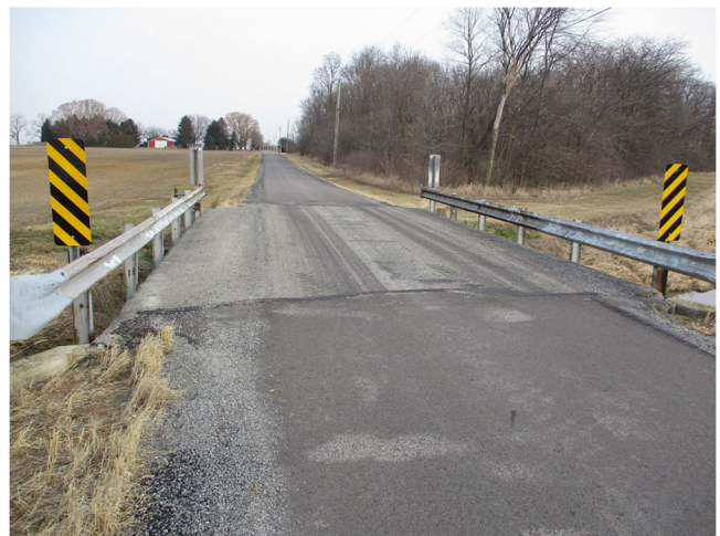
Portage TR 137 Bridge Replacement
