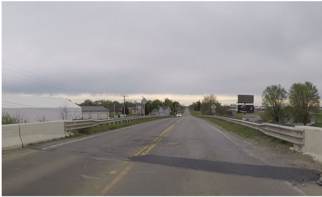
County Road 313 - Prior to Resurfacing
