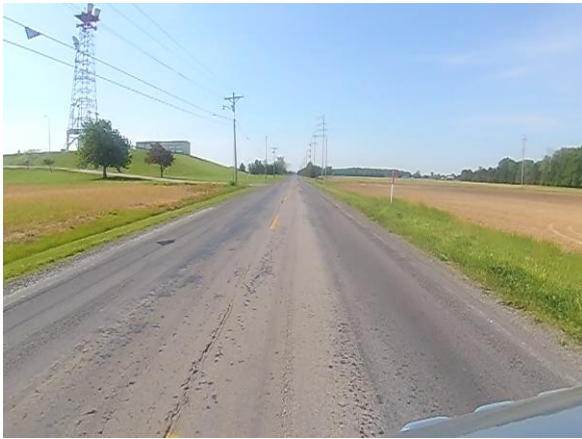
County Road 16 – Before Resurfacing
