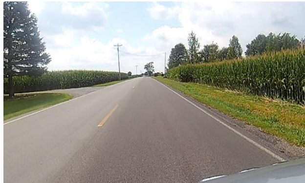
Left Lane – Untreated, Right Lane - Replay BioSpan Replay Asphalt Sealer
