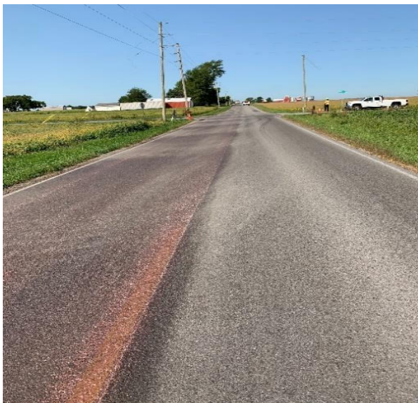
Left Lane – Reclaimite, Right Lane - Untreated Reclaimite Asphalt Rejuvenator
