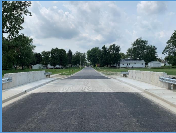
Location: Howard St over Howard Run Between Broad Ave & Fox St
