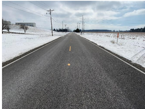
County Road 16 – After Resurfacing
