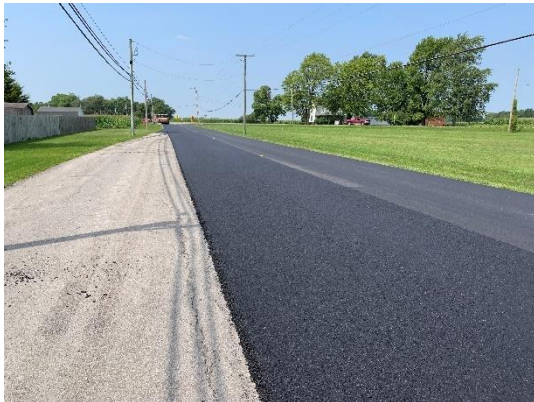
County Road 88 – During Resurfacing
