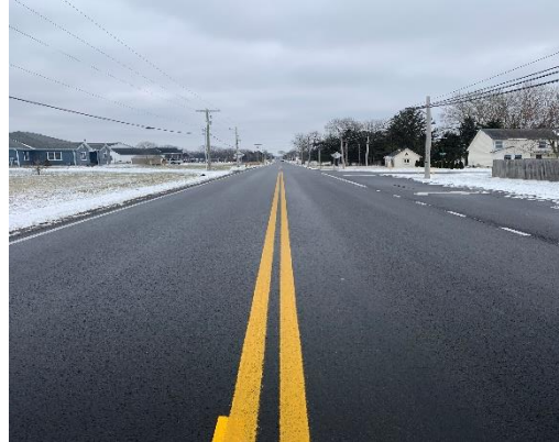
County Road 88 – After Resurfacing
