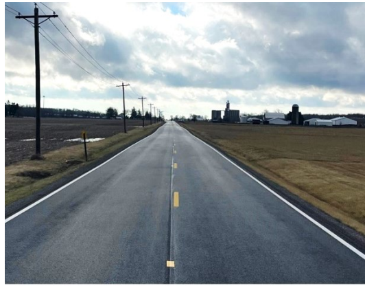
County Road 236 – After Resurfacing
