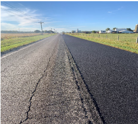
County Road 236 – Before Resurfacing
